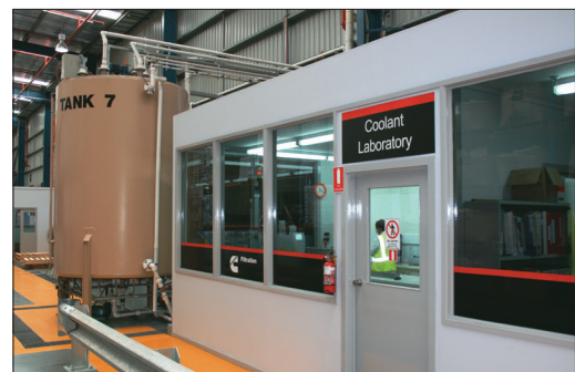
Fig. 1 Cummins Filtration's coolant facility in Melbourne
